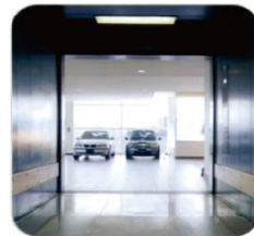
⌘ Front-and-rear opening elevator car
